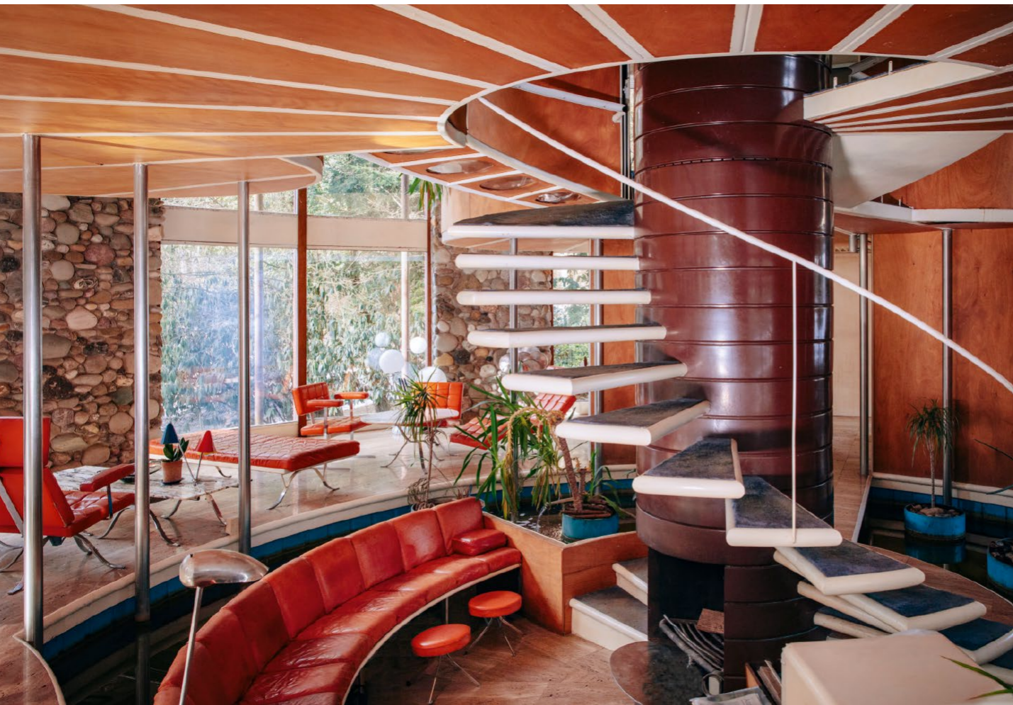
The steel spiral staircase forms the main core of the building. It is one of Otto Kolb’s most important inventions
