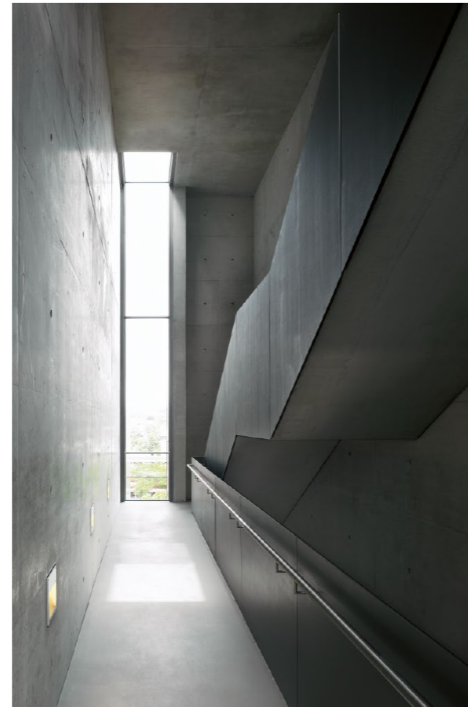
Sleek: the concrete in the stairway glows in the light from the ribbon windows with such silky-smoothness that you almost want to stroke it
