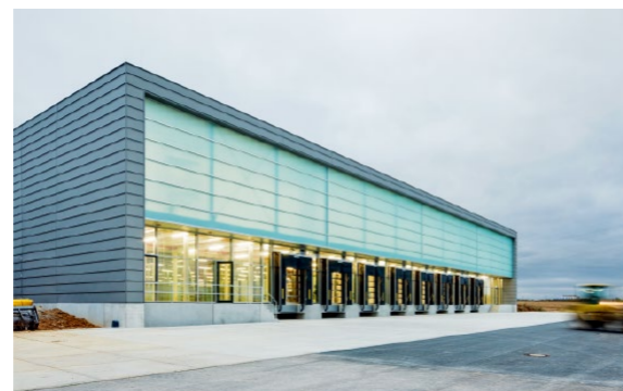
Corporate architecture: the factories in Mötzingen are built around the idea of a brace surrounding a transparent cube
