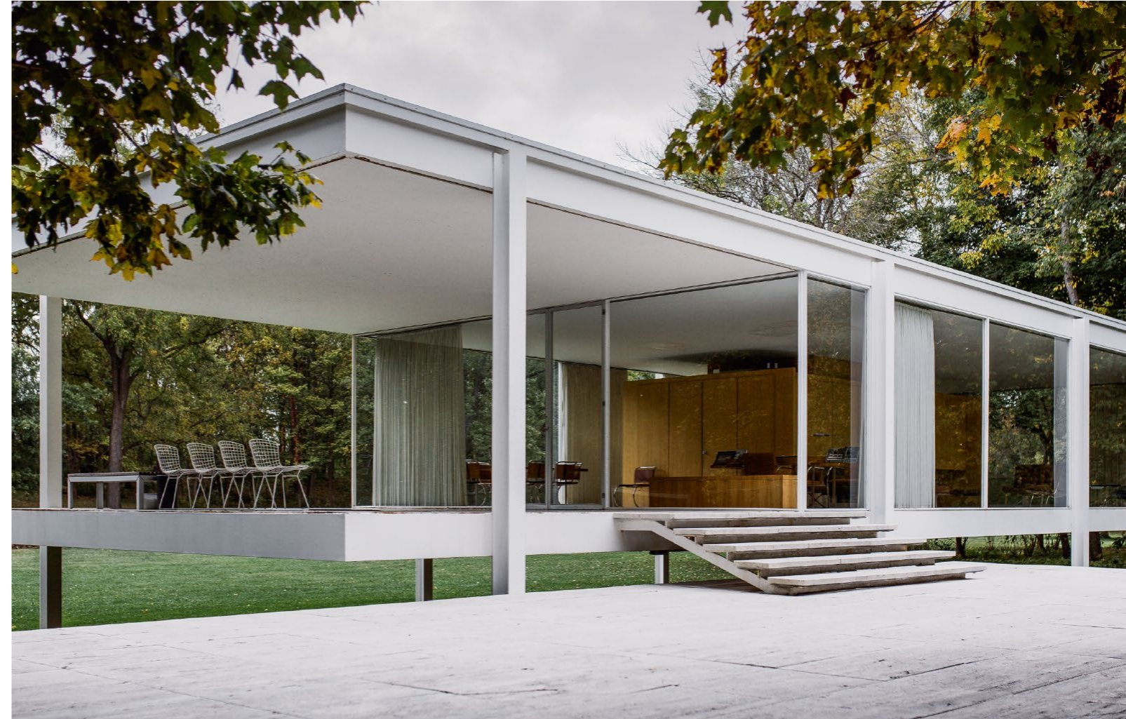
Mies van der Rohe selected only the finest materials: Roman travertine slabs, primavera wood and sandblasted steel
